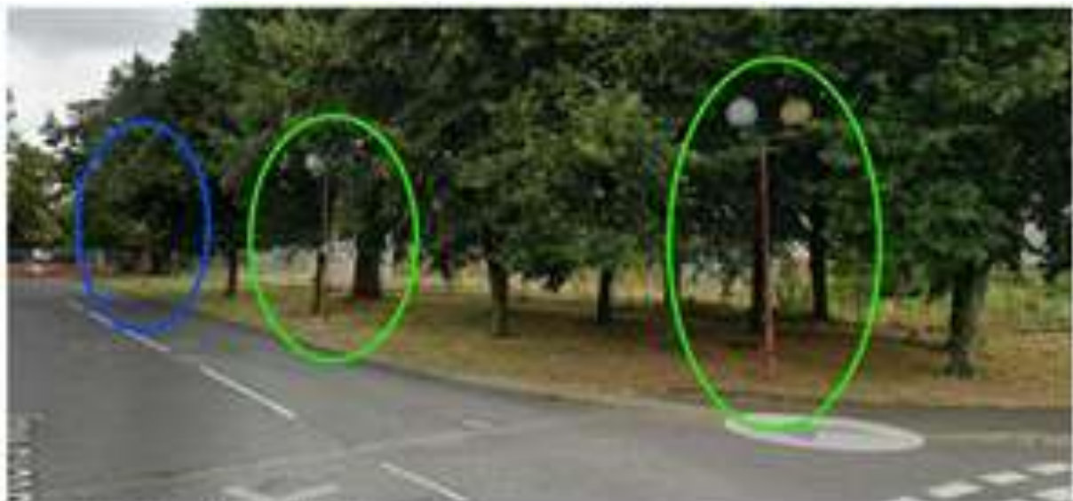
Existing Lighting Columns, Foresters Way Stub
