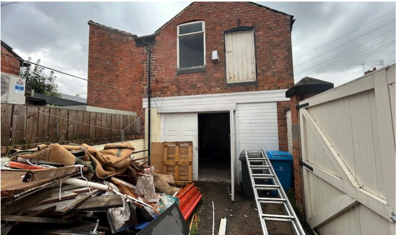
Figure 1: Existing building and yard
