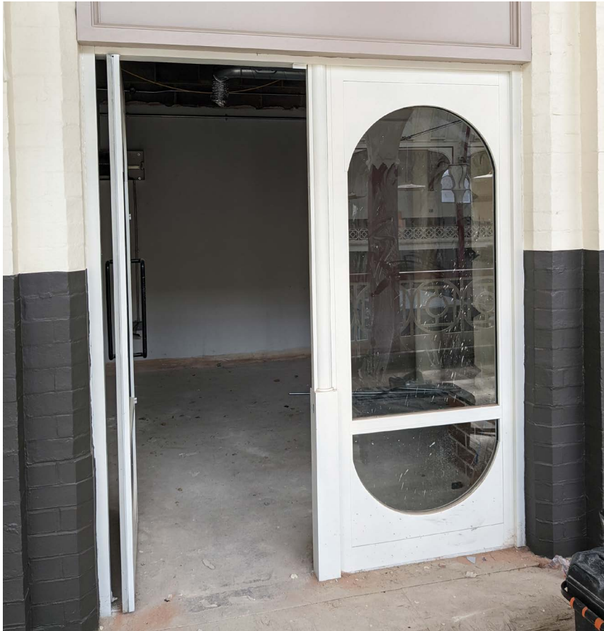
Fig. 3: Existing door - typical photo
