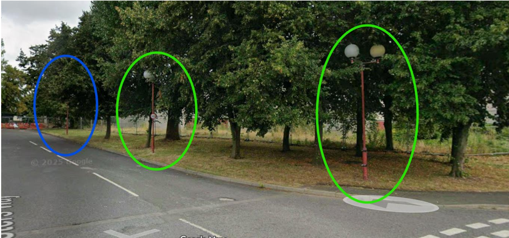
Existing Lighting Columns, Foresters Way Stub
