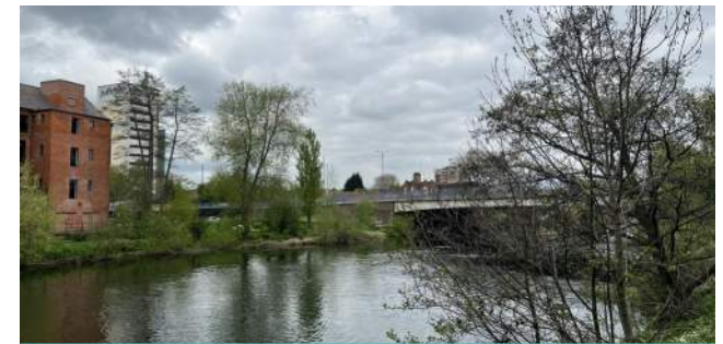
Looking towards Causey Bridge
