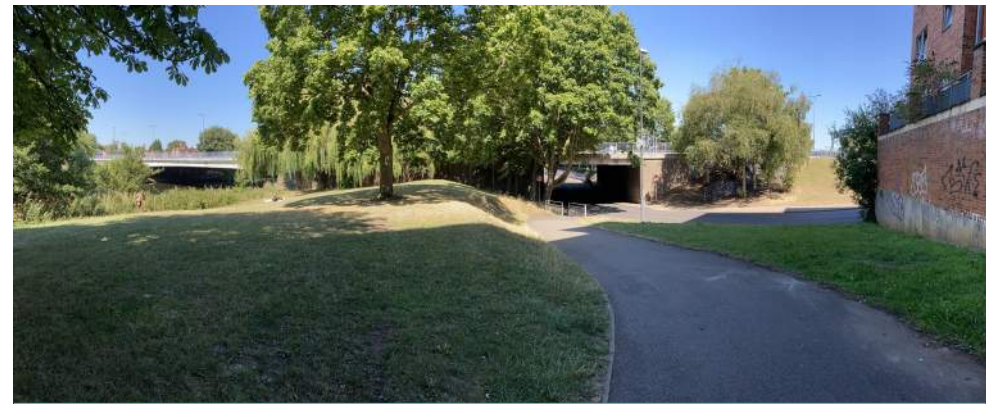
Existing Flood Defences: Reach 1
