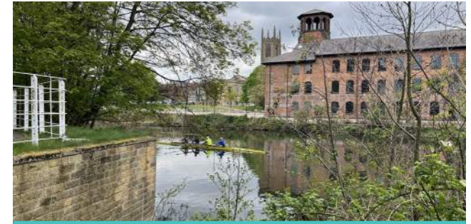
View from north-western corner of Site
