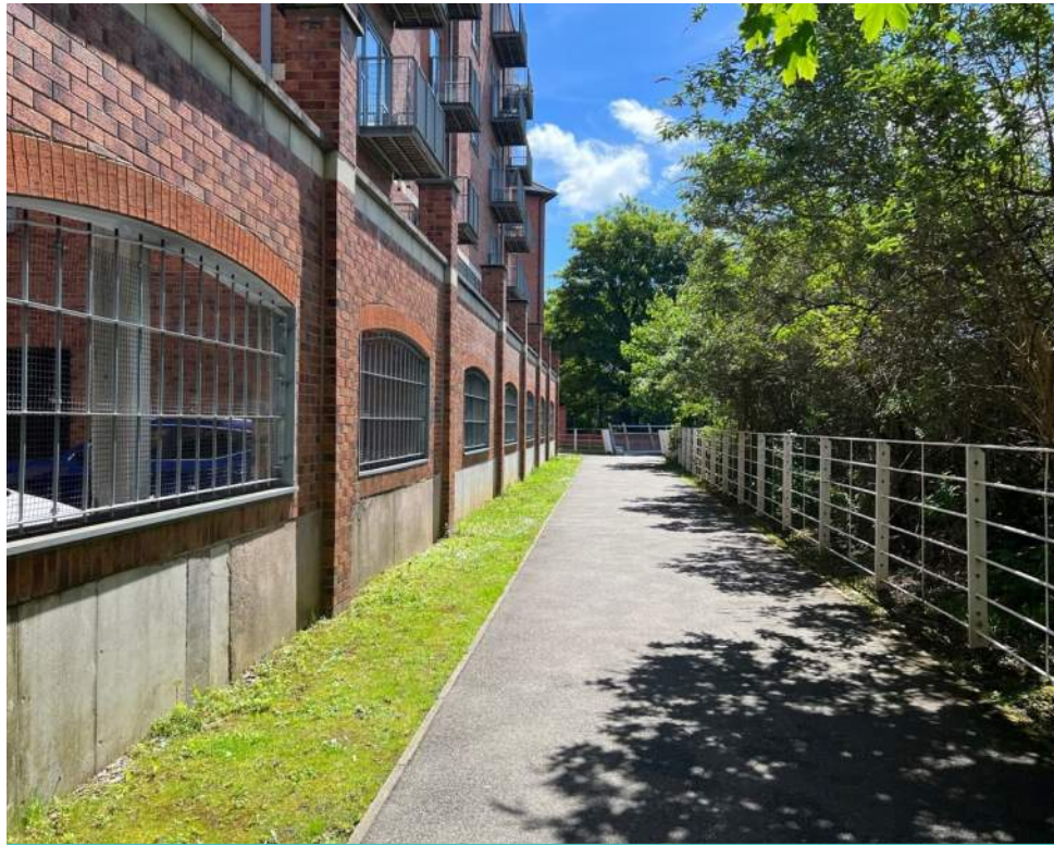
Existing Flood Defences: Reach 2
