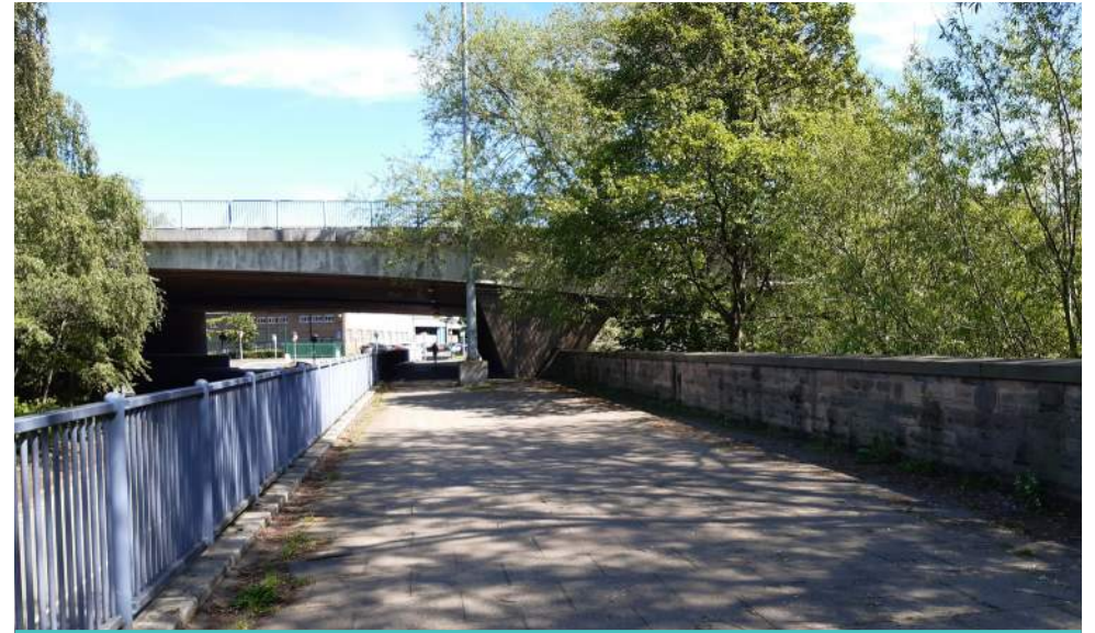
Existing Flood Defences: Reach 5
