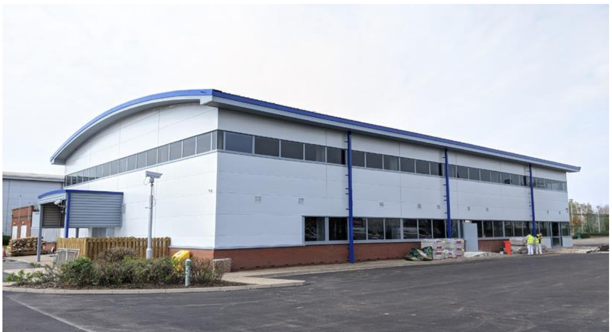
Figure 4 – The Orbis building prior to the flues and chimneys being added
